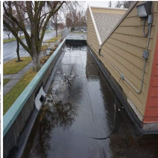
Photo 3 - Standing Water on Roof
