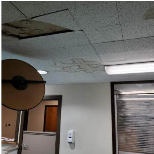
Photo 2 - Water Damage to Ceiling Tiles
