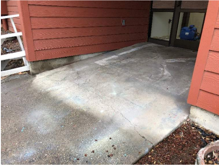
Steep Slope @ Exit Door
