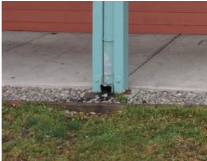
Photo 4 - Water Collection at Base of Columns
