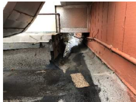
Photo 4 - Standing Water @ Built-Up Roofing
