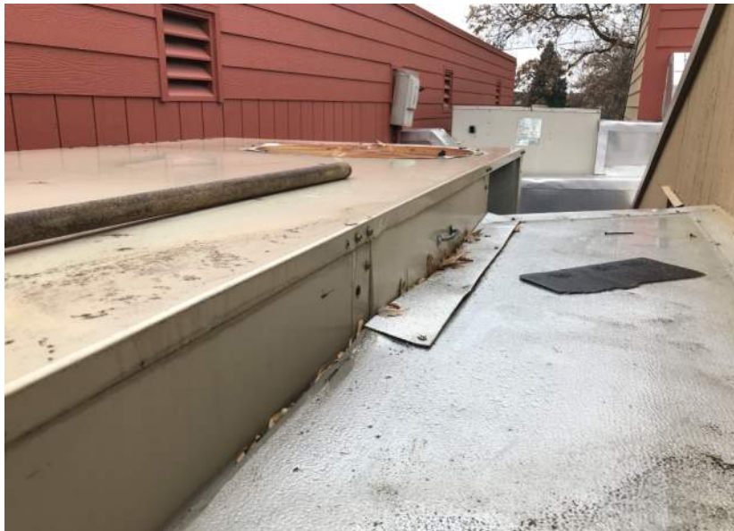
Photo 3 - Access to air filter is blocked by duct insulation. Seam between air handler and duct insulation is not watertight.
