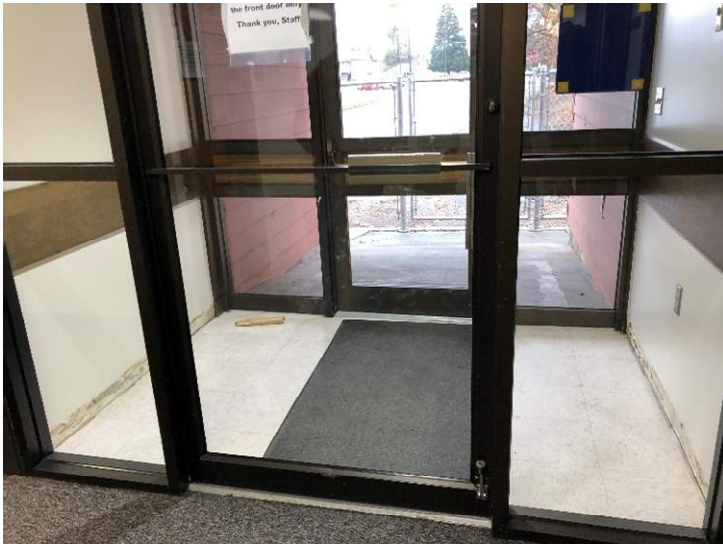
Double Cylinder Deadbolt @ Exit Door
