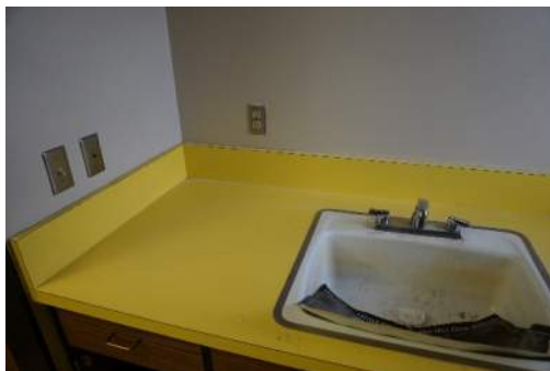
Photo 1 – GFCI Outlets Missing
