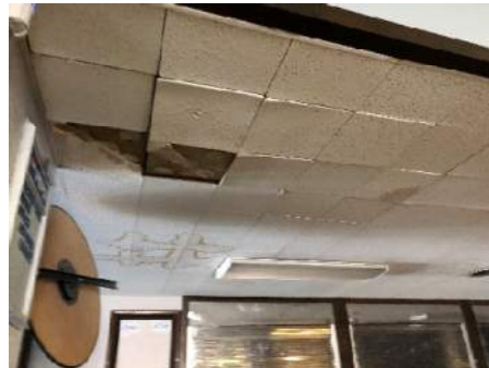
Photo 12 – Water Damage @ Boxing Gym Entry
