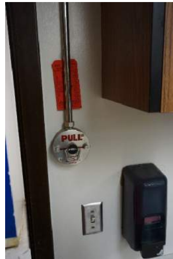
Photo 7 – ANSUL System Manual Activation Station
