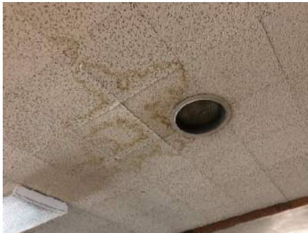
Photo 11 – Water Damage @ Corridor
