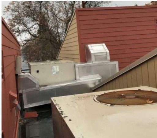
Photo 2 - Rooftop air handling units are difficult to access on the flat section of roof.
