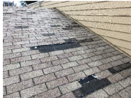
Photo 2 - Missing Shingles
