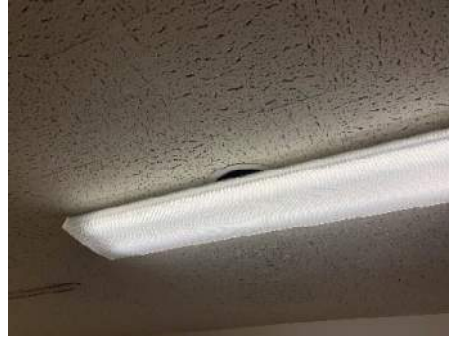
Photo 10 – Replacement Light Fixture Over Can Light
