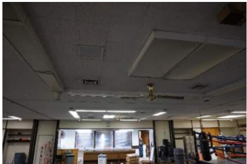
Photo 3 – Existing T8 Light Fixtures
