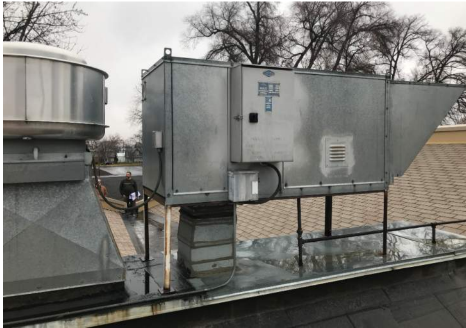
Photo 5 - Kitchen hood exhaust fan and makeup air unit on roof.
