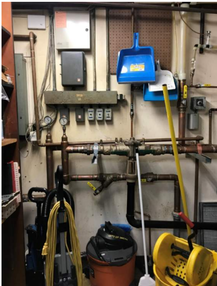
Photo 1 - Domestic water backflow preventor located in the Janitor's closet.
