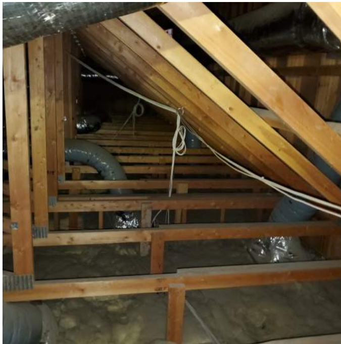
Photo 1 - Typical Truss Roof
