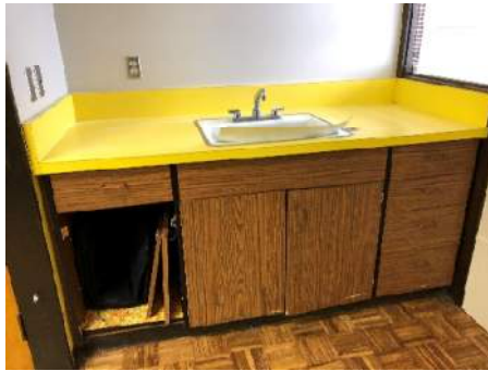
Photo 7 – Casework in Poor Repair
