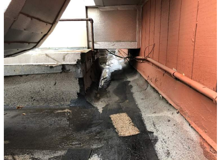
Ponding @ RTU Curbs
