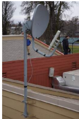
Photo 9 – Satellite/Airpipe Internet System
