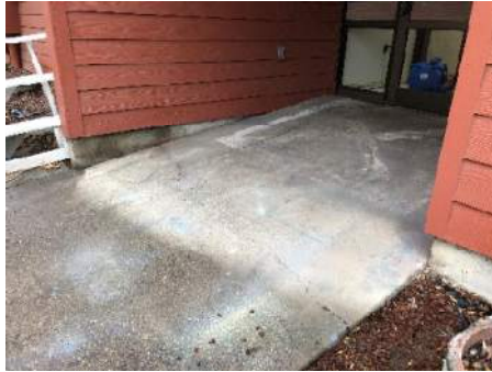
Photo 5 – Excessive Slope @ Egress Door
