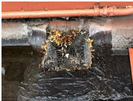
Photo 3 - Poorly Detailed Roof Drain
