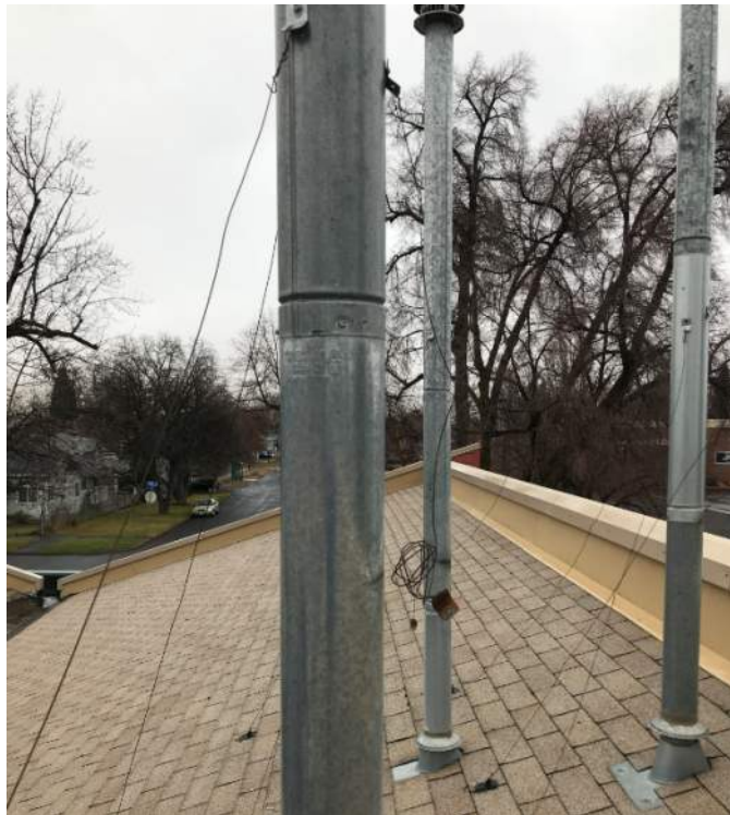
Photo 4 - Guy wires for the furnace and water heater flues have been disconnected from the roof cap.
