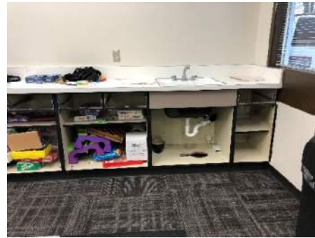
Photo 8 – Casework in Poor Repair
