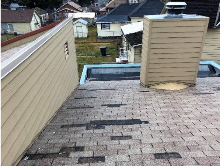
Missing Shingles @ Roof
