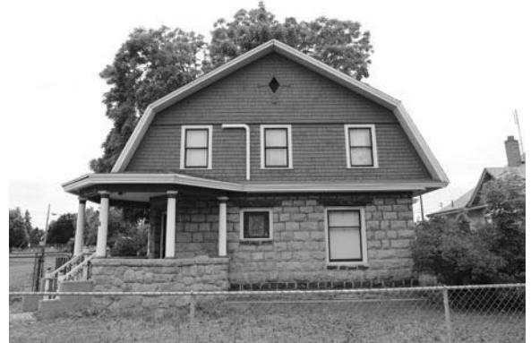
Figure 14. Gambrel Roof Example. 602 North Naches Avenue (ca. 1901), front east facade.
