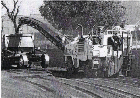
Asphalt grinding – exposing base of road
