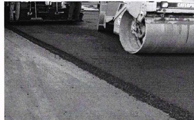
Overlay of a "lift" of asphalt
