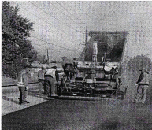
Applying asphalt
