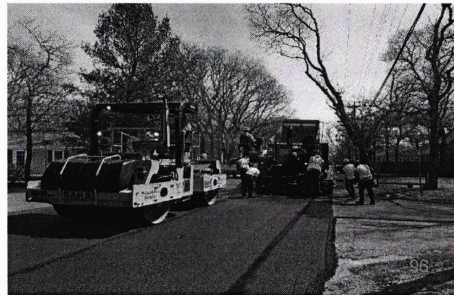
Compacting the aggregate into the oil with a roller
