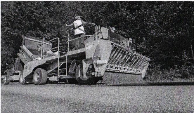
Chip spreader applying crushed aggregate
