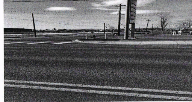
New sidewalks with ADA ramps
