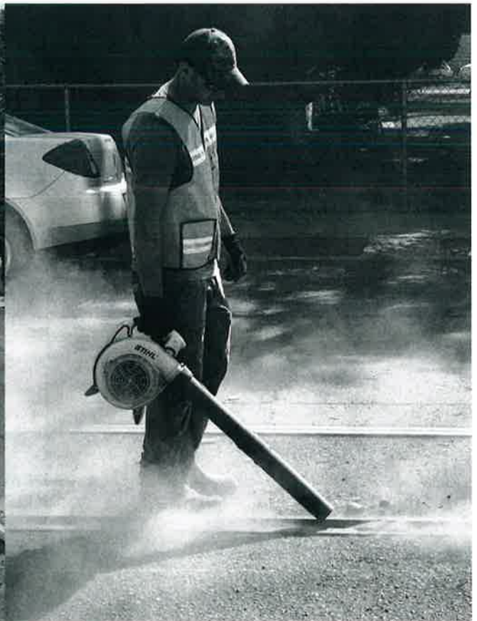
ONE OF THE TREETOP EMPLOYEES, MATT COLVIN, USES A WEED BLOWER TO HELP REMOVE THE IMPACTED GRAVEL AND DIRT FROM THE TROLLEYS' FLANGWAY
