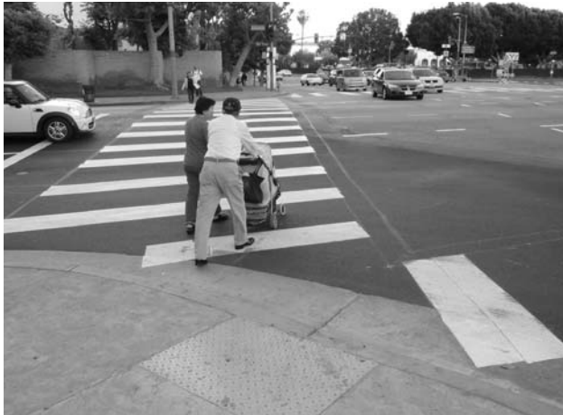
Not recommended: Diagonal curb ramp configuration.
