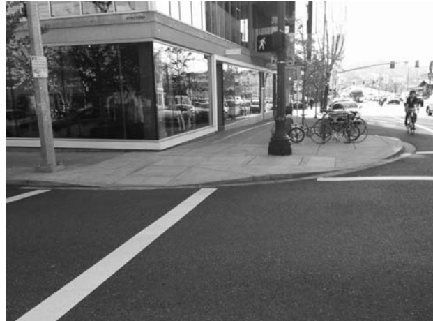
Recommended: Curb extension with bidirectional curb ramps for crossing in both directions.
