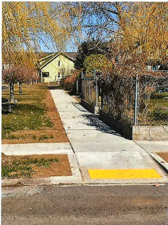
Completed sidewalks with ADA ramps on 4 th St.
