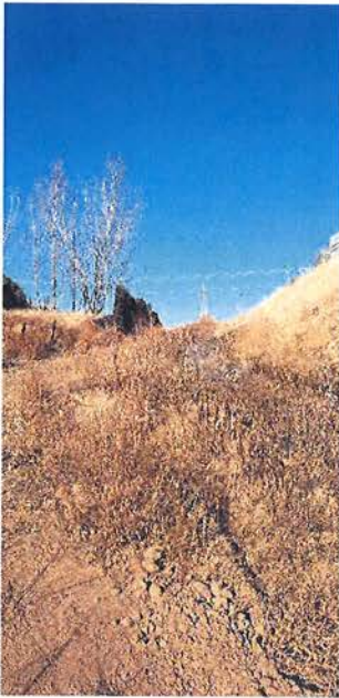
Photo 5. Drainage Path Down Easement
