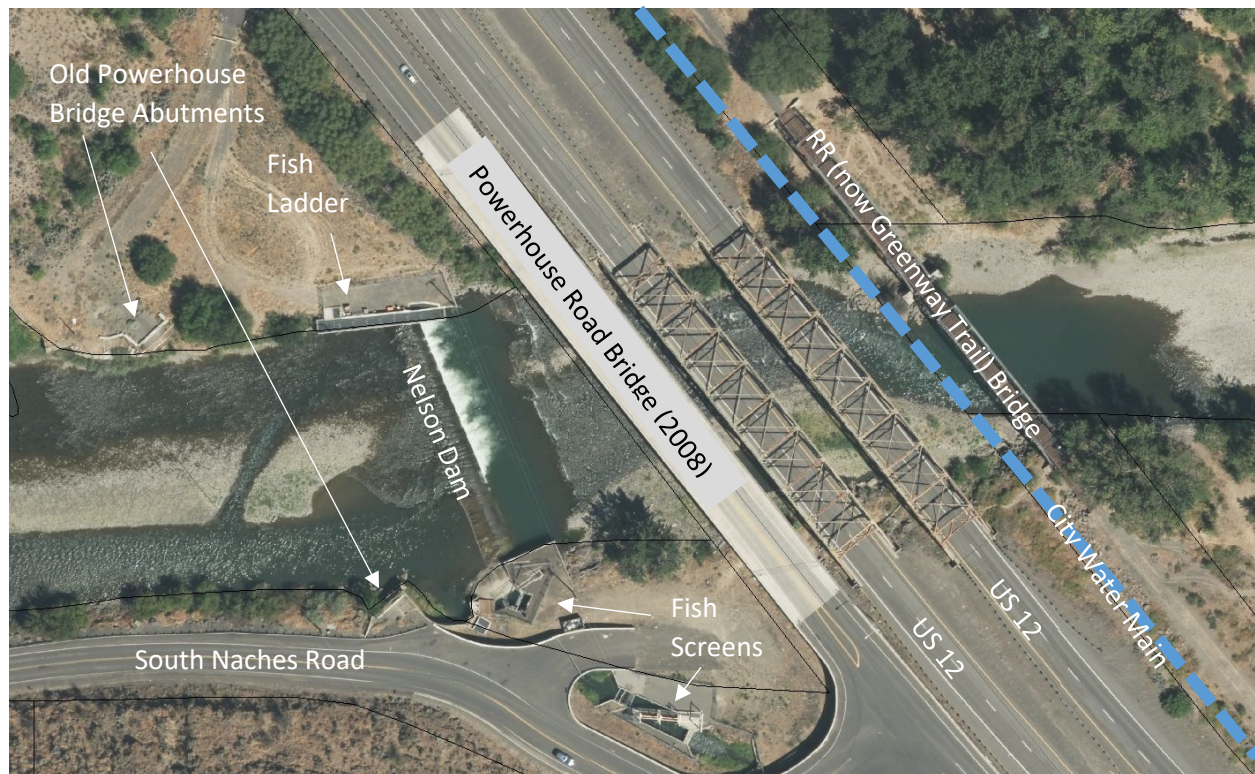
Figure 9 – Aerial view of Nelson Dam vicinity with infrastructure labeled. The photo was taken during the very low flow of summer 2015. Note that the river tends to hug the Tieton Andesite wall near S. Naches Road, which provides good flow to the irrigation diversions and fish screens, but poor flow to the fish ladder. Note channel cut across bar to improve flow to the ladder.
