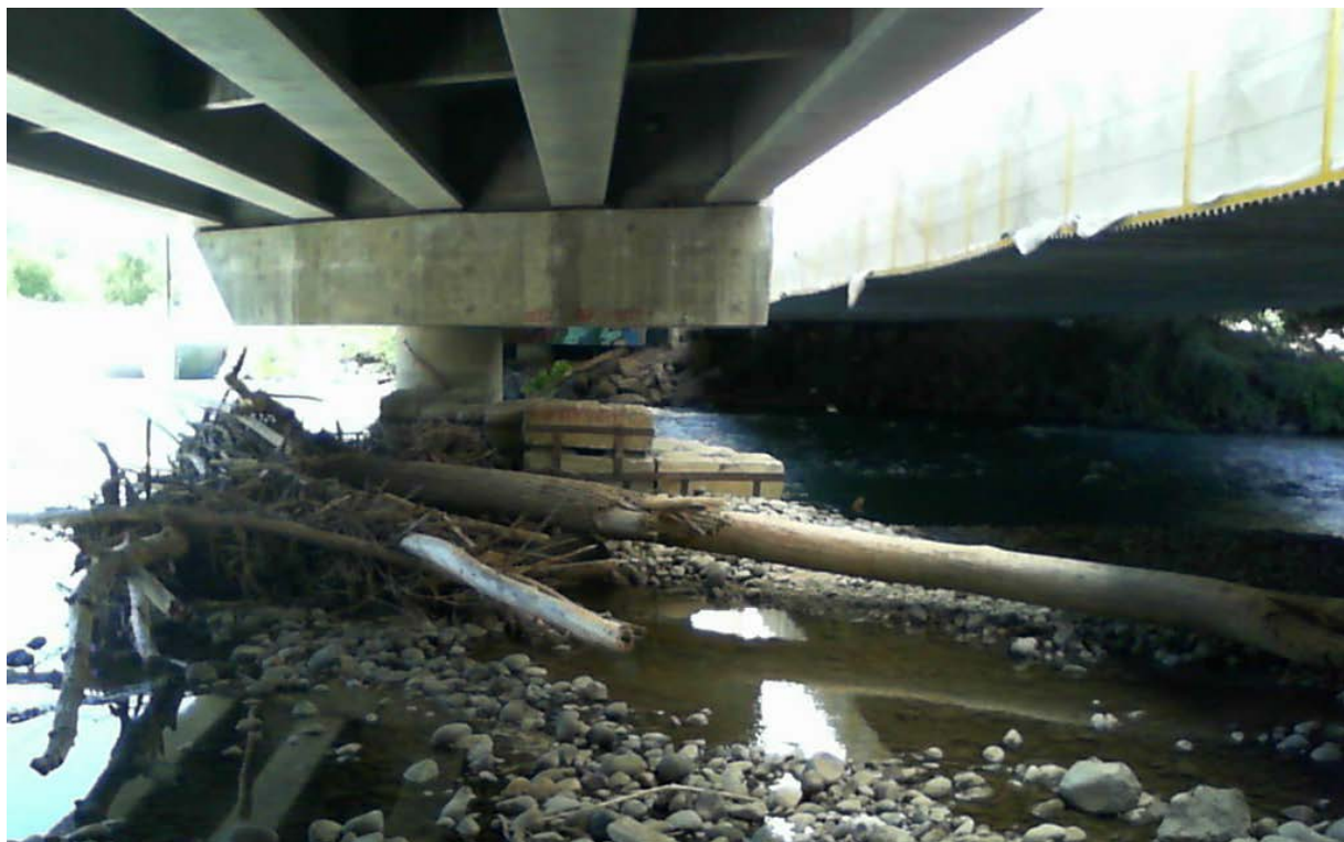
Figure 11 – Fish bypass discharge pipe location beneath Powerhouse Road Bridge. “Ecology Block” structure and racked woody material shown. (downstream US 12 bridge is sheathed in plastic for painting)
