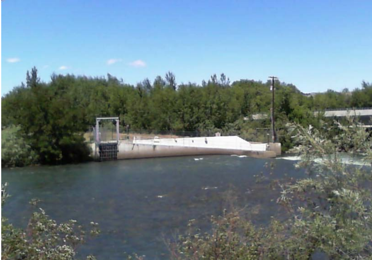
Figure 10 – Fish Ladder Entrance at Nelson Dam, 2018
