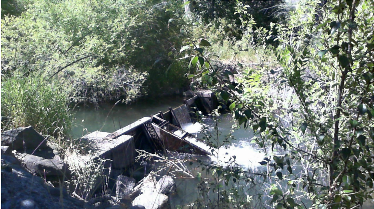
Figure 15 – Dam and Fishway at Cowiche Creek mouth.
