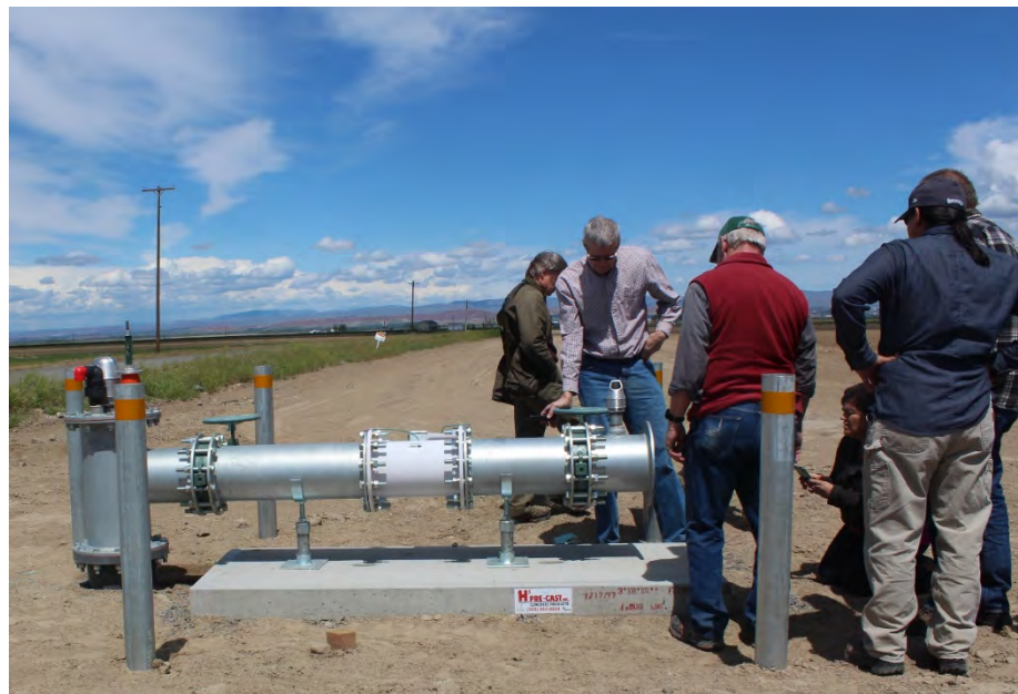
WIP Infrastructure Improvements
